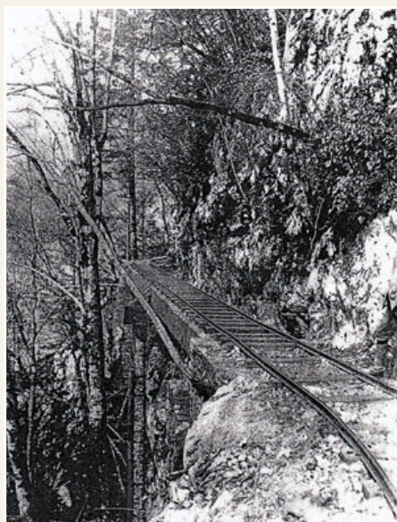
Wooden bridge («mostovž») on the route of the narrow-gauge motor-powered railway in Strug
