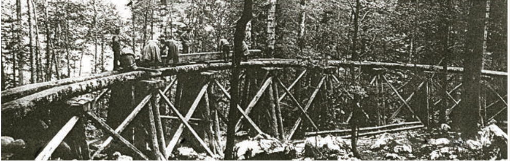
Construction of the wooden trestle bridge ("veksl") where the line of the motorised narrow-gauge railway turned towards Idrija
